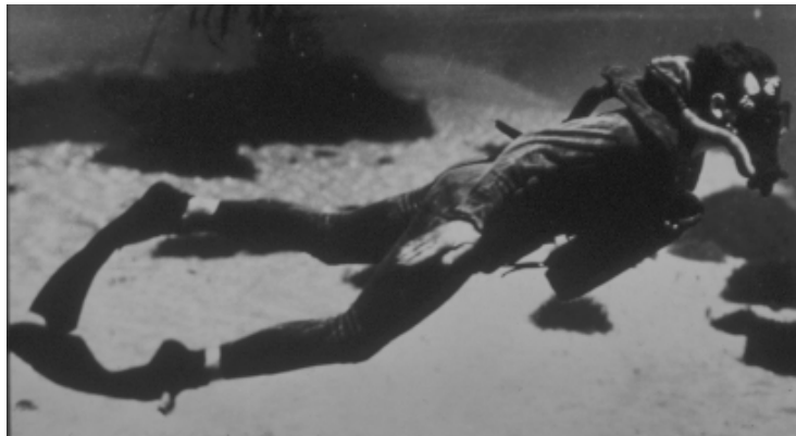
Exhibit Fig 1. An Office of Strategic Services (OSS) swimmer is pictured underwater using the Lambertsen Amphibious Respiratory Unit (LARU) Mark 10, also called the Lambertsen rebreather, on a training exercise in 1943. Photograph: Courtesy of C. J. Lambertsen, Philadelphia, Pa.
